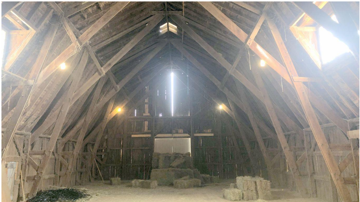
Caption: Photograph of interior of Hayloft in OAC barn (1). Taken at Guelph University.
